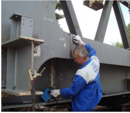
Ultrasonic testing in site of welds of bridge elements
